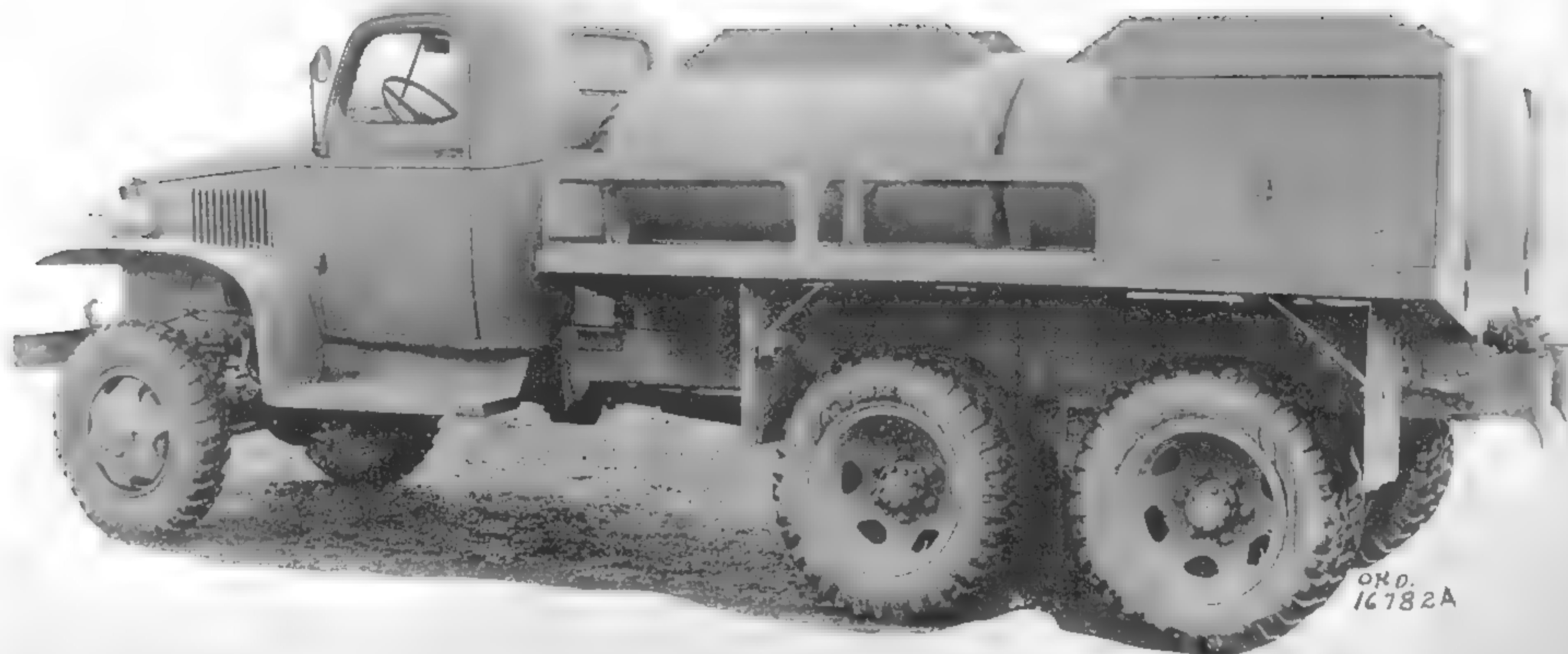
This 1942 photo of a closed-cabbed fuel tanker truck was taken at Holabird, Maryland. The bed actually houses two separate fuel tanks. The racks alongside the tanks were used to store auxiliary fuel cans. (National Archives and Records Administration photo)
